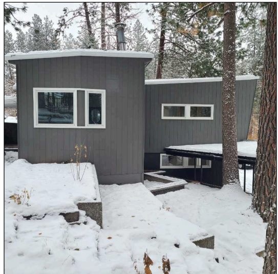
West side of home.
